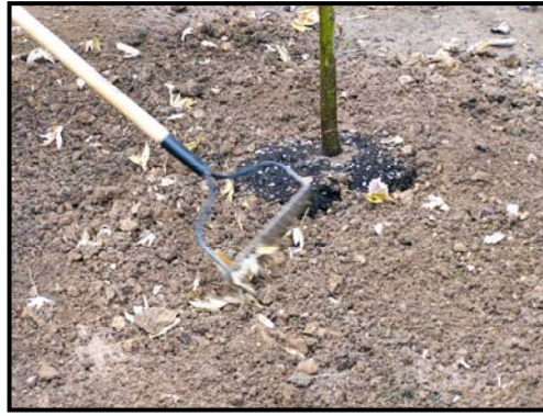
Figure 27. Final grade. Note how the root ball soil is visible on the surface, with no backfill covering the top of the root ball.
