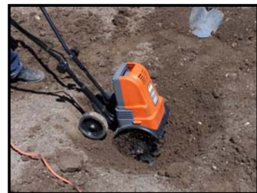
Figure 16. Digging the hole with a small tiller or "garden weeder."
